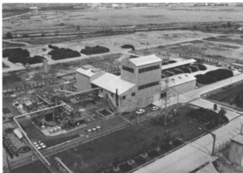
Figure 4. View of the actual plant
