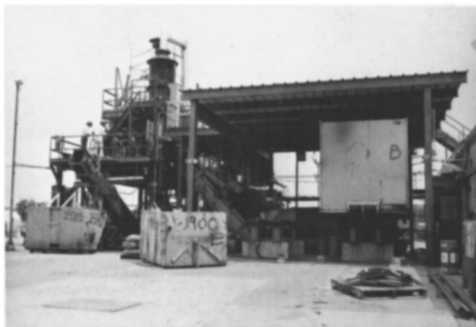
Figure 3. Overall view of the pilot plant
